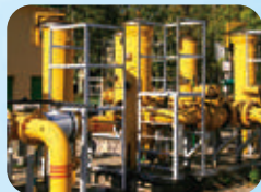
Storage Tank Monitoring
