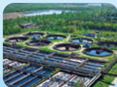
Water Treatment Plant System
